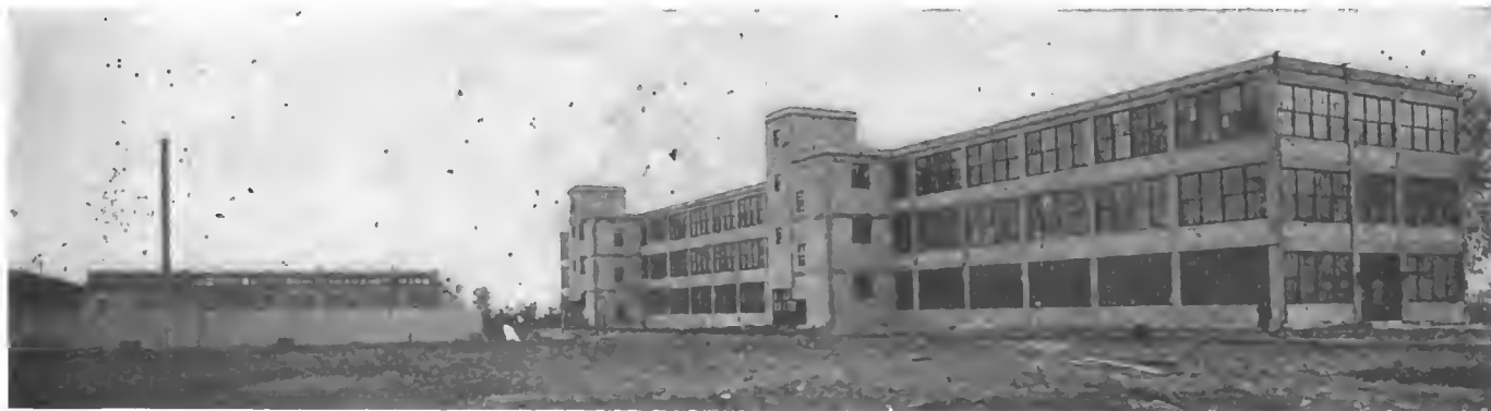
NEW REINFORCED CONCRETE FIREPROOF FACTORY OF THE E. R. THOMAS DETROIT COMPANY, ON JEFFERSON AVE., DETROIT.
